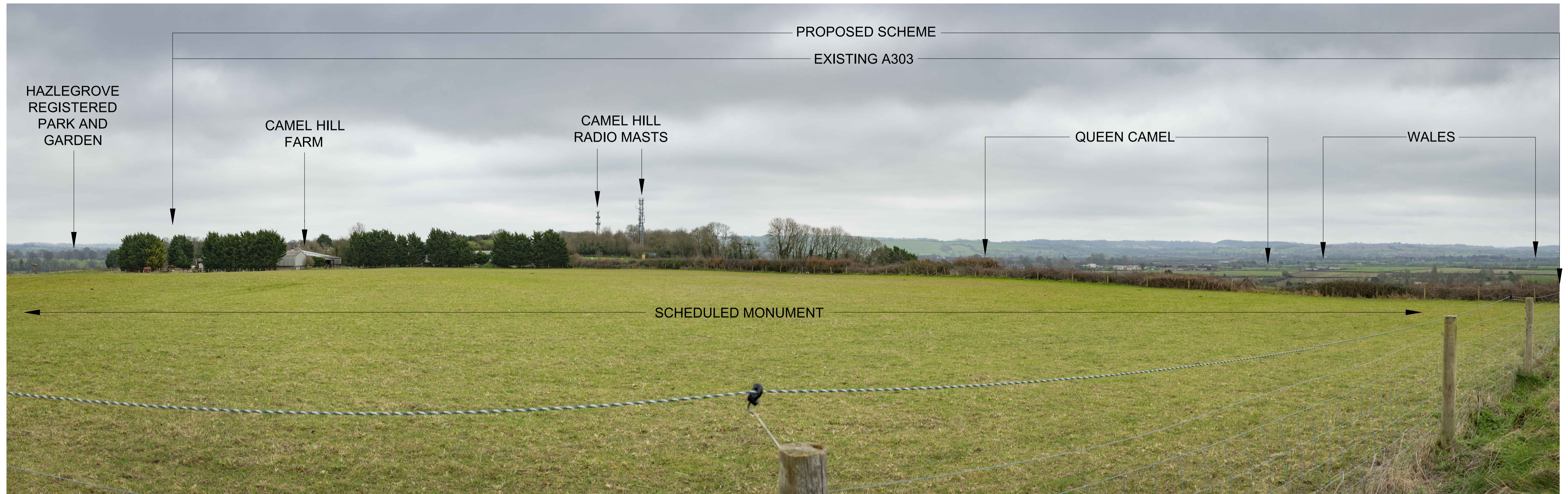
EXISTING VIEW LOOKING SOUTHEAST TOWARDS EXISTING A303 REPRESENTATIVE OF CAMEL HILL FARM SCHEDULED MONUMENT, APPROXIMATELY 80m FROM SCHEME.
